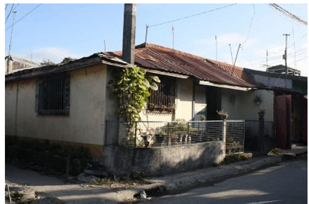
FRCB's Church Building in Muzon, Bulacan
